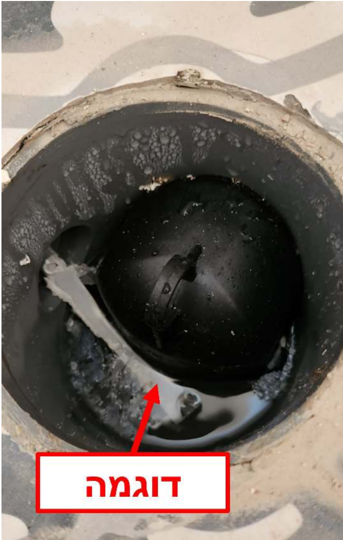
a) Floor gully with side inlets and flange for bonding membranes (example)
